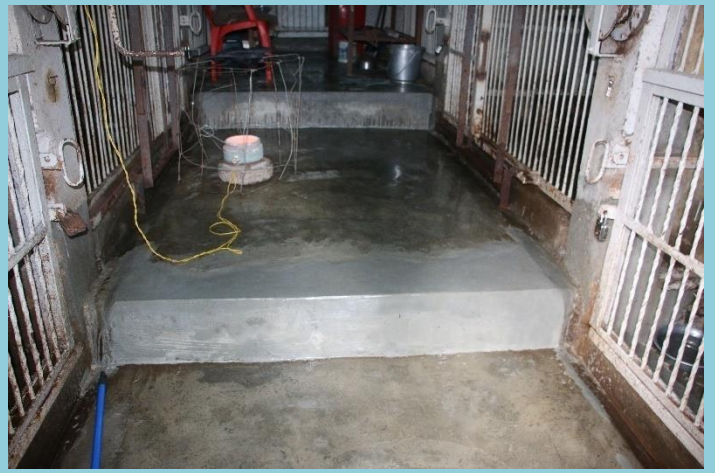
Repair of the keepers resting room and night shelters
