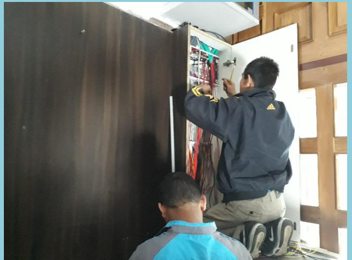
Electrical work at BNHM
