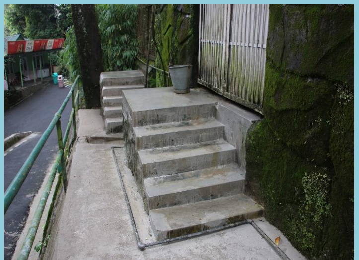
Repair of stairs leading to the night shelter of Black leopard
