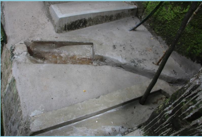
Repair of drains in the night shelters
